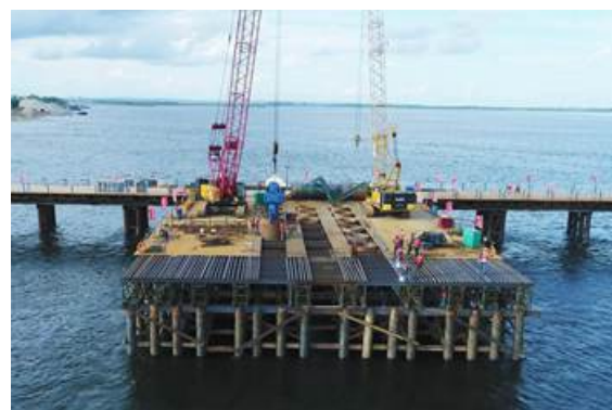
Road bridge linking NE China and Russia under construction
